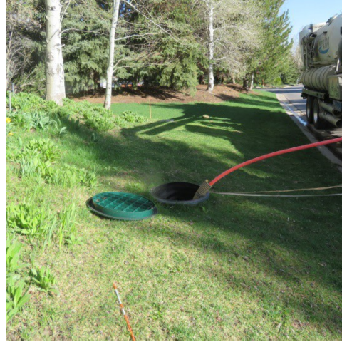
Mh 6A Pro-Pipe clean-out through to Willow Creek.
