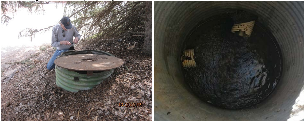
Clay measuring height of water in steel conduit. Height of water less than 6". Damage to tubes.
