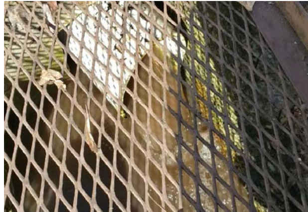
Segment A's only discharge drain; via Mh 6A outlet through solid PVC discharge pipe in easterly direction, under E. Meadows Drive, between Lot 105 & 106, into Willow Creek. This drain is the only place where the UD water reaches full Daylight.
